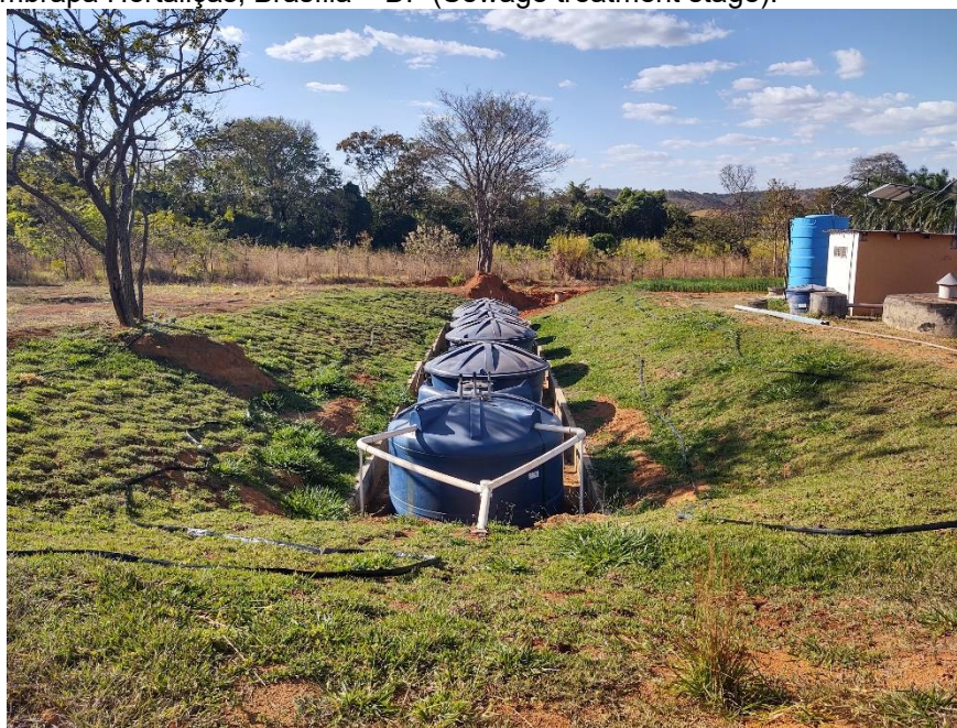
Figure 2 – Prototype of the ReAqua System to serve about 300 people operating under operational conditions (TRL/MRL 6) at Embrapa Hortaliças, Brasília – DF (Sewage treatment stage).
